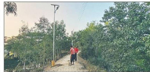
A solar street light being set up along a road in Kultali in the Barulpur subdivision of South 24-Parganas
