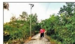
The street lights being installed
